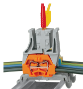
Testing after the conductors have been terminated.
