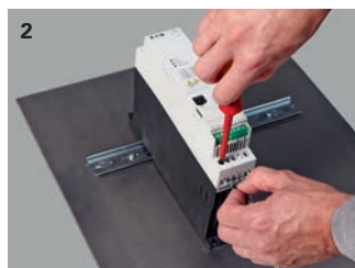
2 Connect mains and motor cables.
