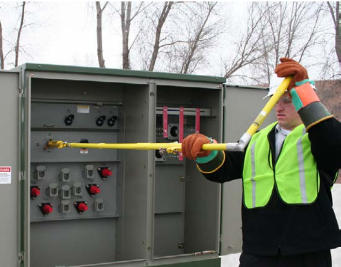
18-inch fit-on leverage tool provides mechanical advantage during loadbreak switching
