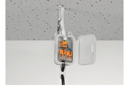
Pendant light connection in a suspended ceiling
