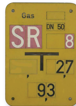
Information on location of gate valve
