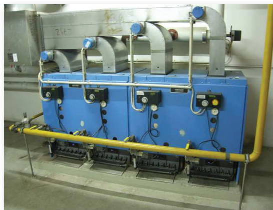
Atmospheric 4-stage gas boiler
