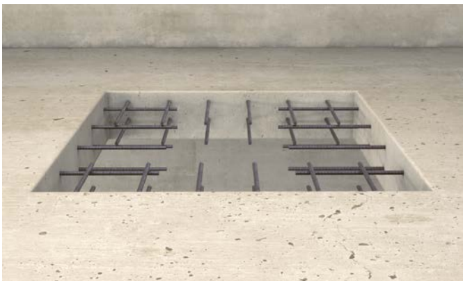
Closing a ceiling opening
