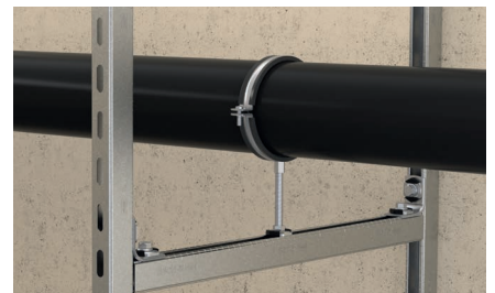
Horizontal pipeline on frame construction
