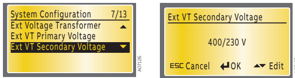
Figure 7.16 Ext VT Secondary Voltage, factory setting is 400/230V
