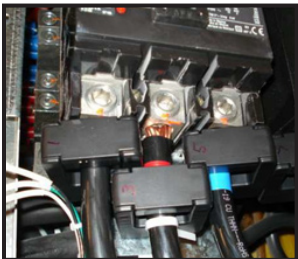
Figure 8. CT Connection Points (300 A CT Shown)
