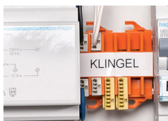
Example of a residential door bell application – carriers mounted on a DIN-35 rail
