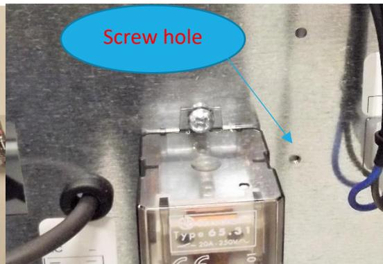
Figure 3: mount here with screws.
