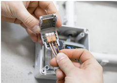
Place the wired connector in the Gelbox.
