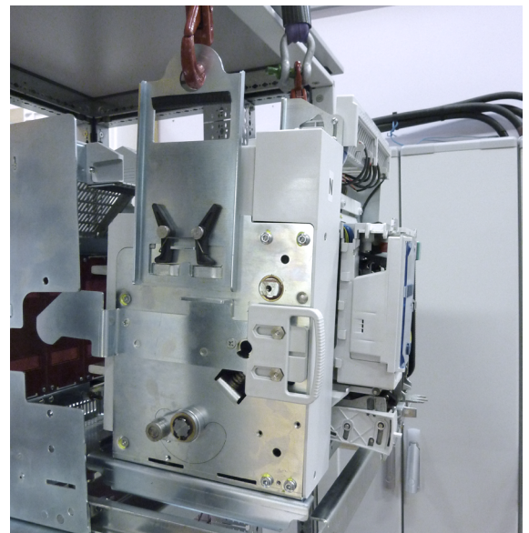
Placement of a draw-out DMX 3 in its base
