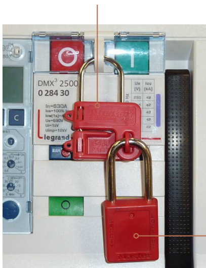
Padlocking the ON and OFF buttons
