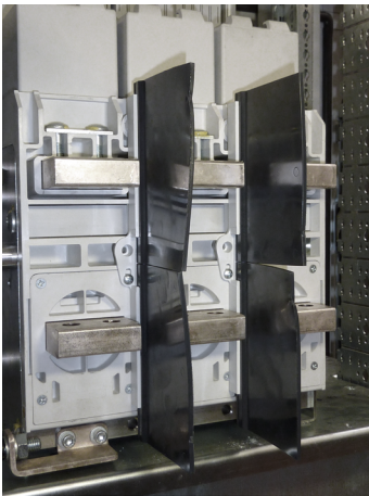
Example : insulated shields mounted on the fixed DMX 3 3P
