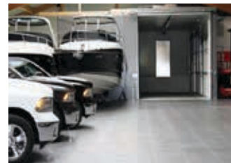
With the goods lift, boats can be transported to the fourth floor – this can now be done by pressing a button on a smartphone
