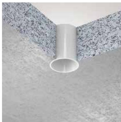
**Fig. 7:** Lost lining in solid ceiling
