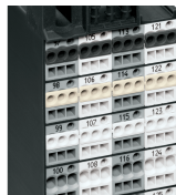
Insulation stop is in place.
