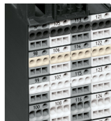
Insulation stop is in place.
