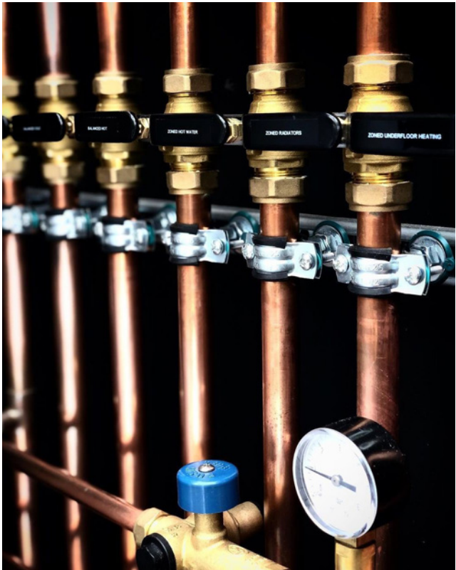
Installation by Glistar Services
