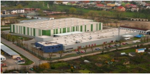
Fig 1. A view of Armacell Poland Sp. z o.o. factory in Środa Śląska (Poland).
