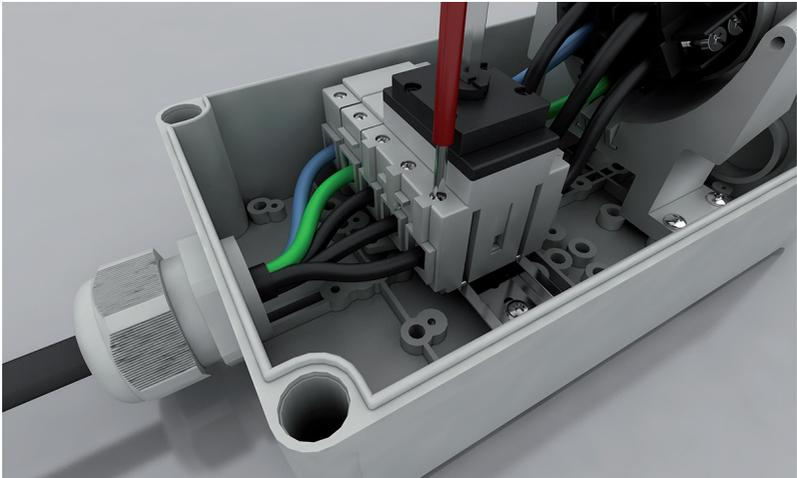
8. Check whether the individual conductors are seated tightly by pulling them lightly. If this is not the case, open the terminal and repeat the previous step.
