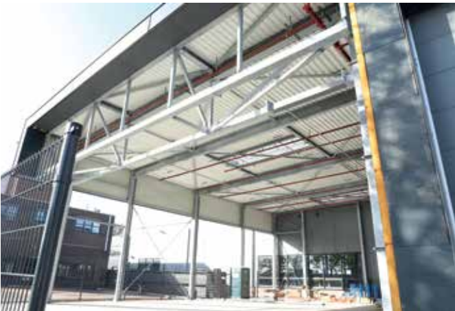
Truck loading dock - The Netherlands
