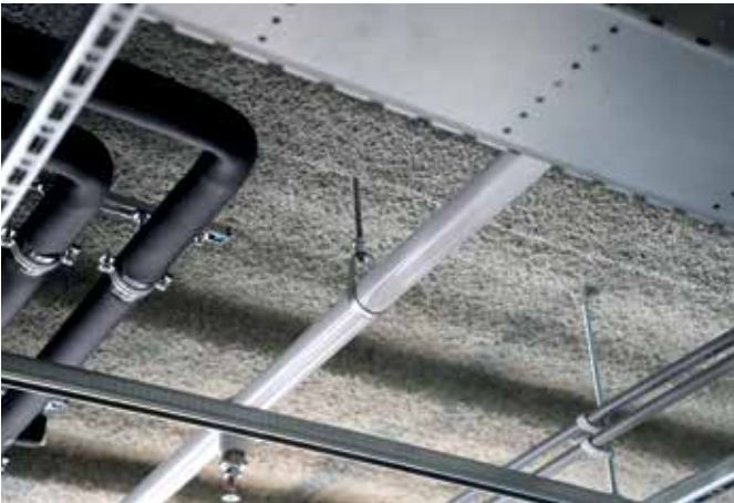
Office building - The Netherlands
