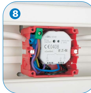
Installation of the actuator in a cable channel box
