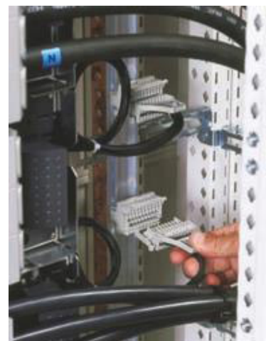
Auxiliary connection block in the connection compartment.
