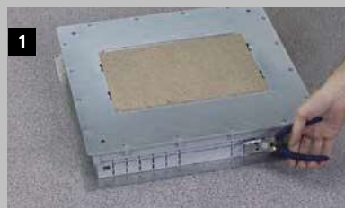
Trim the trunking entries
