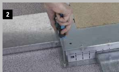
Insert the trunking and screw to the floor
