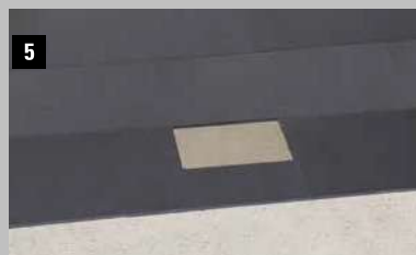
Fit the lining
