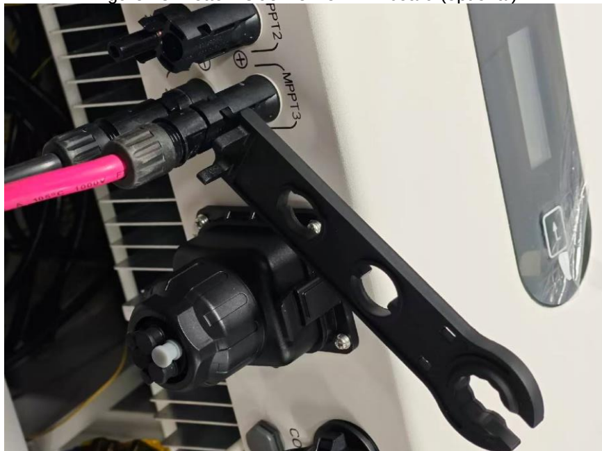
Figure 26. PV connector with tools
