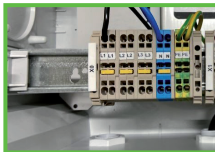
Figure 14 A: 230V connection PURE
