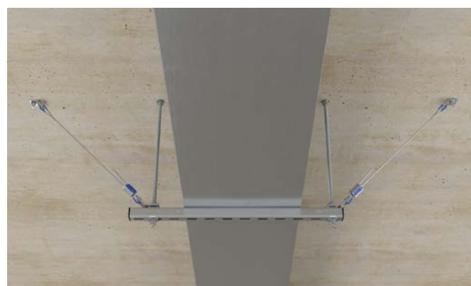
FWI-S Lateral bracing of air ducts
