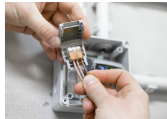
Place the wired connector in the Gelbox.
