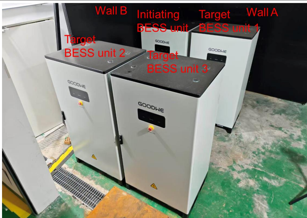
Figure 14. View of initiating BESS unit and target BESS Unit in testing room
