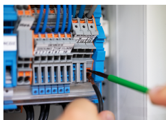
Conductor termination
