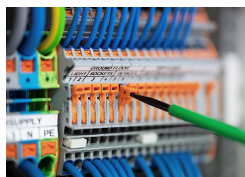
Pivoting a knife disconnect.
