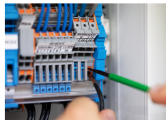
Conductor termination
