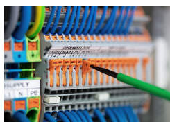
Pivoting a knife disconnect.
