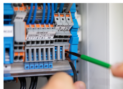
Conductor termination
