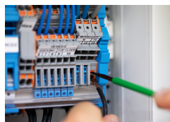
Conductor termination
