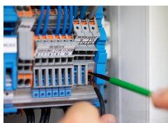
Conductor termination
