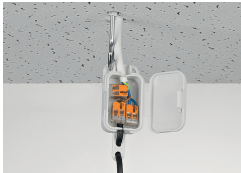
Pendant light connection in a suspended ceiling
