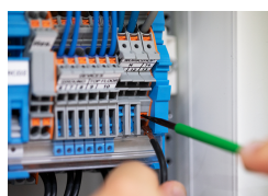
Conductor termination
