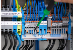
Tool-operated N-disconnect slide link
