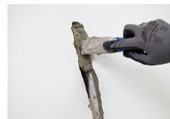
Close the damaged area discreetly.
