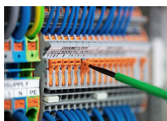
Pivoting a knife disconnect.
