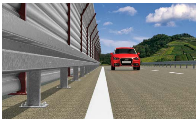
Noise protection walls
