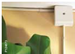
Combined use of clips and Mureva K60 surface-mounted box.
