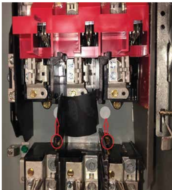
Figure 3. Relocation of fuse clips or fuse bases.
