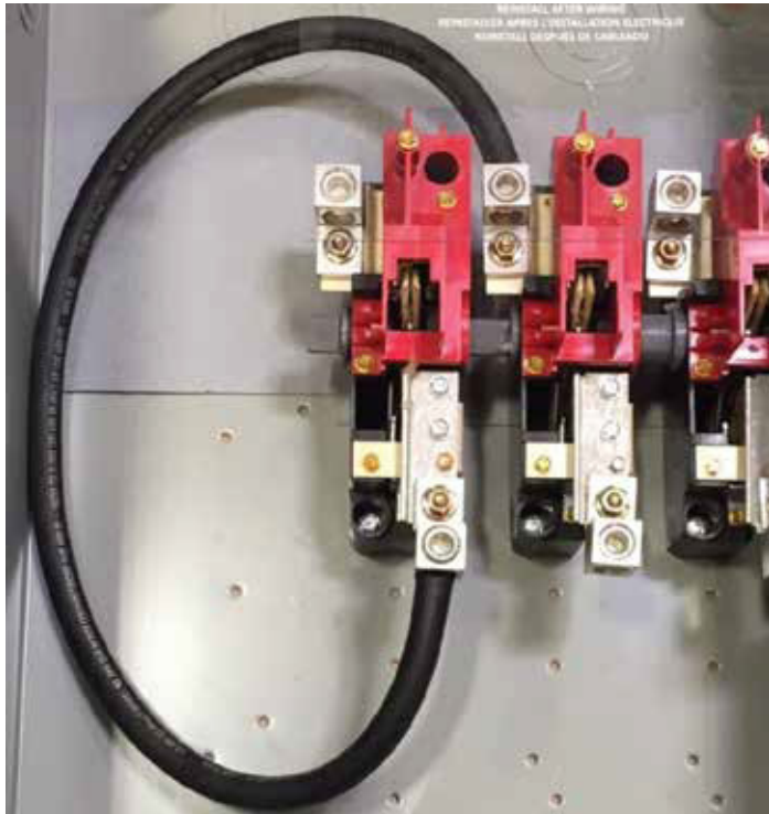
Figure 2. Sample 2-pole 600 V heavy duty safety switch.
