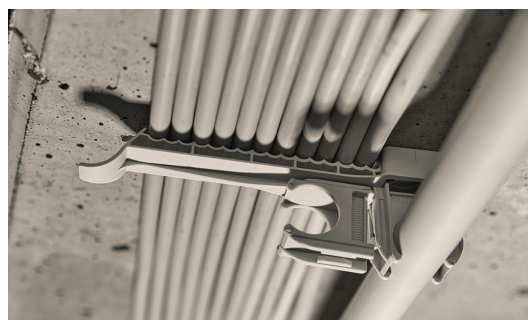
An additional EC Euro-Clip for Pipe installation can be mounted at the center of the KBS.
